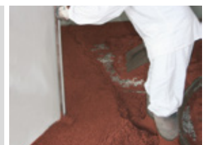
Pour screed (or mortar) into the pockets, compact, and level off.
